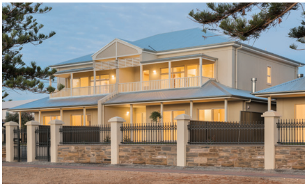
EXCELLENCE IN MEDIUM DENSITY OVER 5 DWELLINGS AREA Construction PROJECT Largs Bay
