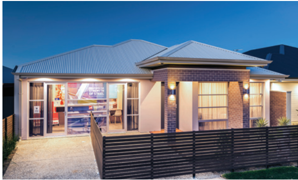
EXCELLENCE IN A DISPLAY HOME UP TO $180,000 WEEKS & MACKLIN BUILDING GROUP PROJECT The Avanti, Penfield
