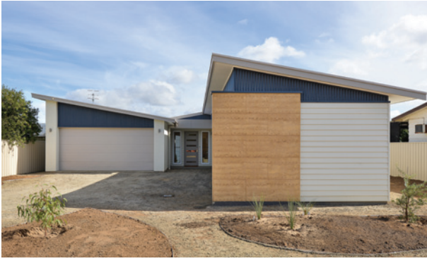
EXCELLENCE IN A CONTRACT HOME $300,000 TO $500,000 SOUTH COAST CONSTRUCTIONS PTY LTD PROJECT Port Elliot
