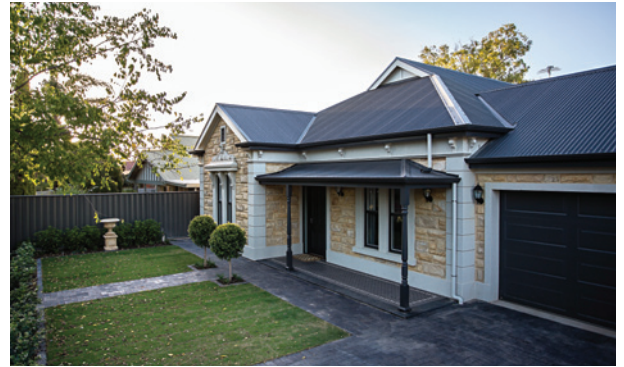
EXCELLENCE IN A CONTRACT HOME $300,000 TO $500,000 CAMPOREALE AND KLEMM BUILT PROJECT Nailsworth
