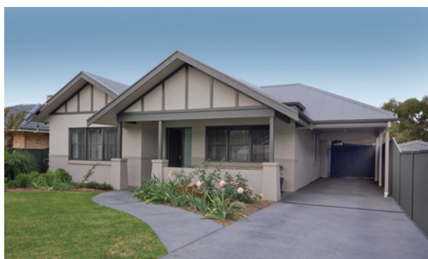
EXCELLENCE IN A RENOVATION OR ADDITION UP TO $200,000 SCOTT SALISBURY HOMES PROJECT Henley Beach
