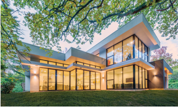
EXCELLENCE IN A CONTRACT HOME $500,000 TO $700,000 SCOTT SALISBURY HOMES PROJECT Stirling
